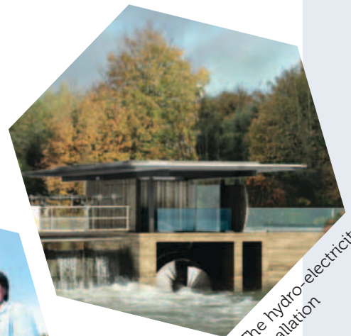
Construction begins on the weir
